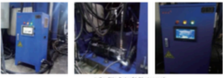
On-Site Retrofit Photograph
