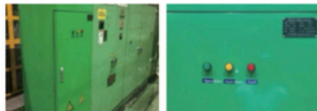
On-Site Retrofit Photograph
