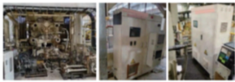
On-Site Retrofit Photograph
