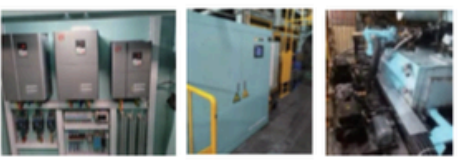
On-Site Retrofit Photograph
