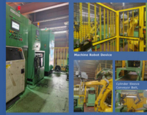
Control Cabinet Device
